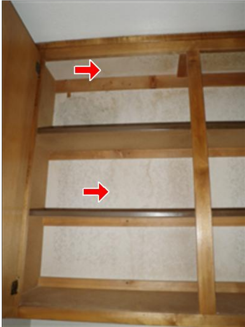
6.2 Picture 1 Hall cabinet next to bath
