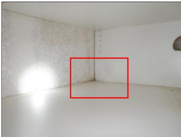
6.6 Picture 2 Left of sink kitchen base cabinet
